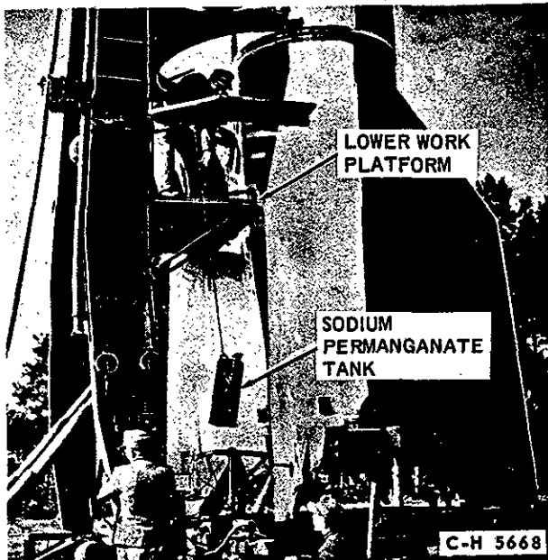
Figure 1-5. Hoisting Sodium Permanganate Tank to Fueling Level
